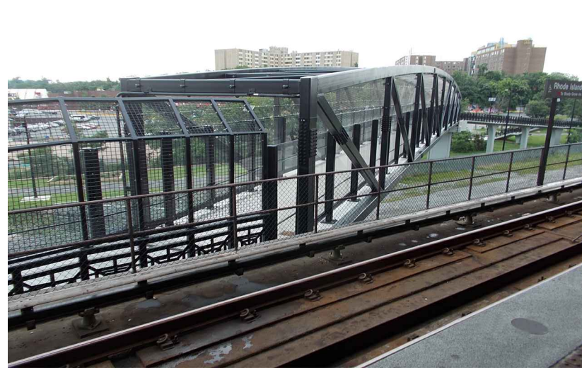
B. Metro Bridge
