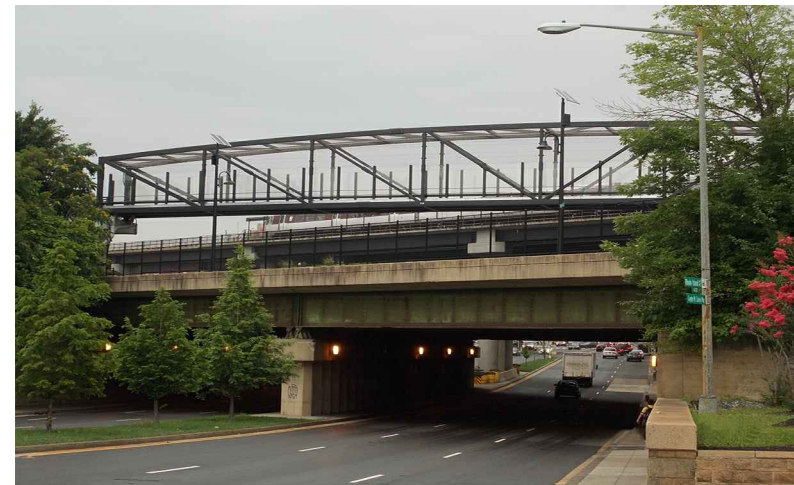
J. Rhode Island Ave. Underpass
